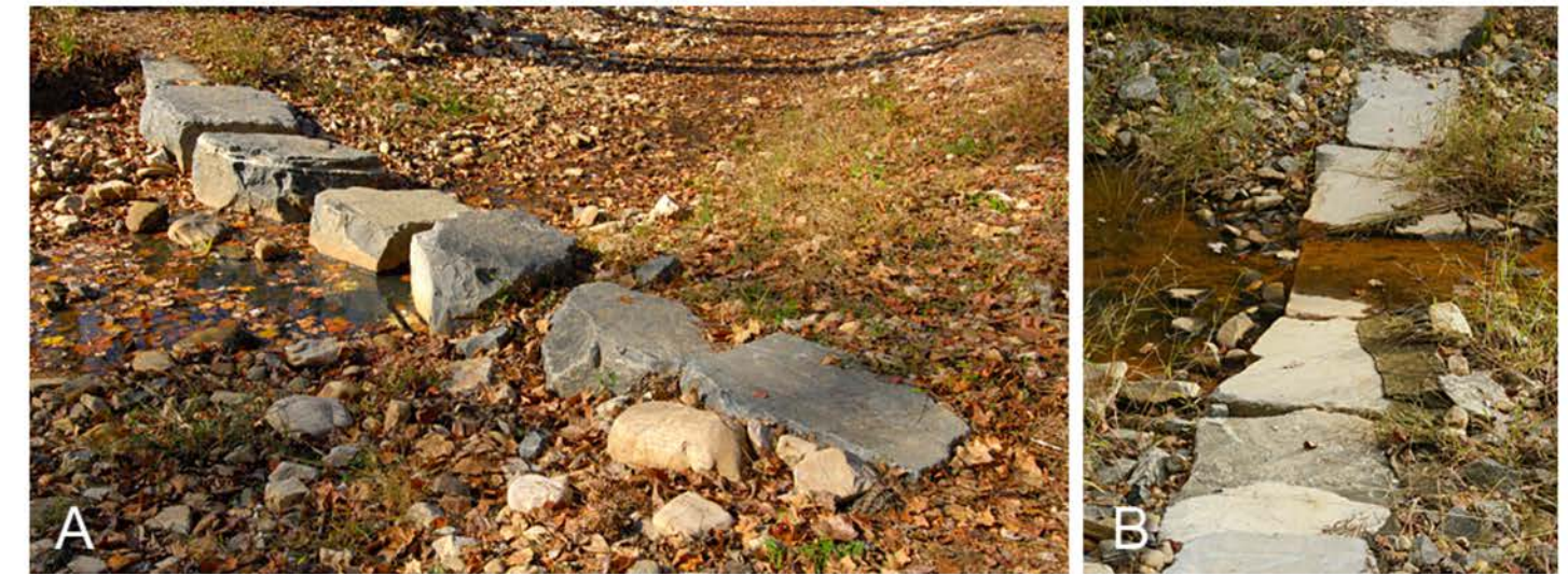
Figure 3. The pre-restoration bridge across Shanes Creek trail was removed. Where trails cross the stream, elevated, fair weather stepping stones are in place (A). Plan your walk accordingly if heavy rain is in the forecast. Carved, partially submerged boulder arrangements called "sills" (B) control the stream. They might look like rustic sidewalks but are not and can be dangerously slippery with algae. Please stay off the sills. Water levels are low in both images due to a drought.
