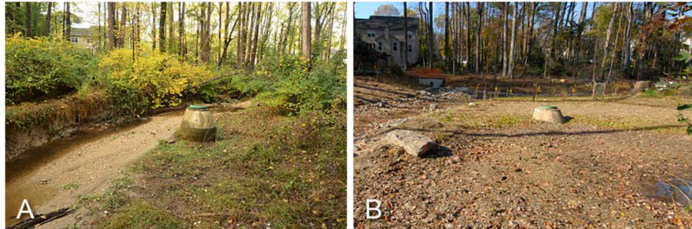
Figure 1. A major factor driving the stream restoration was Shanes Creek's heavily eroded and sunken streambed (A), also seen in some of its tributaries. Years earlier, the creek flowed to the right of the then mostly buried sewer manhole tower. The project elevated streambeds and water tables (B, photographed at the same location after restoration). Some sections were rechanneled. Strategic combinations of stones, logs, and native plants now line and reinforce the streambanks. The concrete-filled, four-inch-diameter PVC tubes are permanent stream stability monitoring stations (C), installed at several places along the restored waterway.
