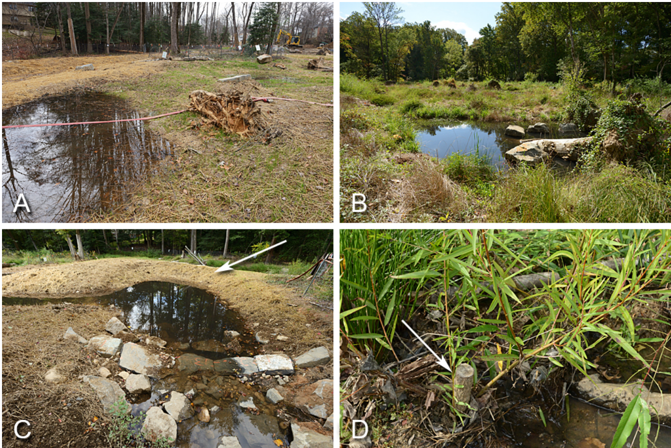
Figure 5. The planners dubbed the project's largest, multi-pooled artificial wetland, "Frog Disneyland" (A, during construction, and B, after). It is 900 feet east of Roberts Road. Instead of being fed by the creek's floods, Frog Disneyland's water comes from a large storm drain outfall—one that was a major source of pollutants entering Shanes Creek and the reason for so much work at this location. After exiting the outfall, water collects in front of a berm (C, arrow) that separates the pool from Shanes Creek before making a 90° turn into the wetland. The plant roots here, including this black willow ( Salix nigra ) sprouting from a livestock in the ground (D), filter pollutants and clean the effluent before it enters the creek. Reducing usage of pesticides and other chemicals that contaminate runoff will improve the environment even more! Frogs are breeding in these artificial depressions as they do in vernal pools . Amphibian populations help gauge a habitat's health because they are sensitive to environmental changes .
