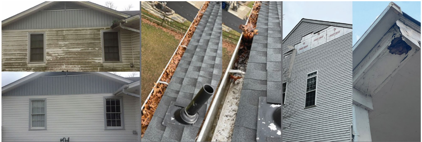
Siding & Trim Repair Rotten Wood Replacement
