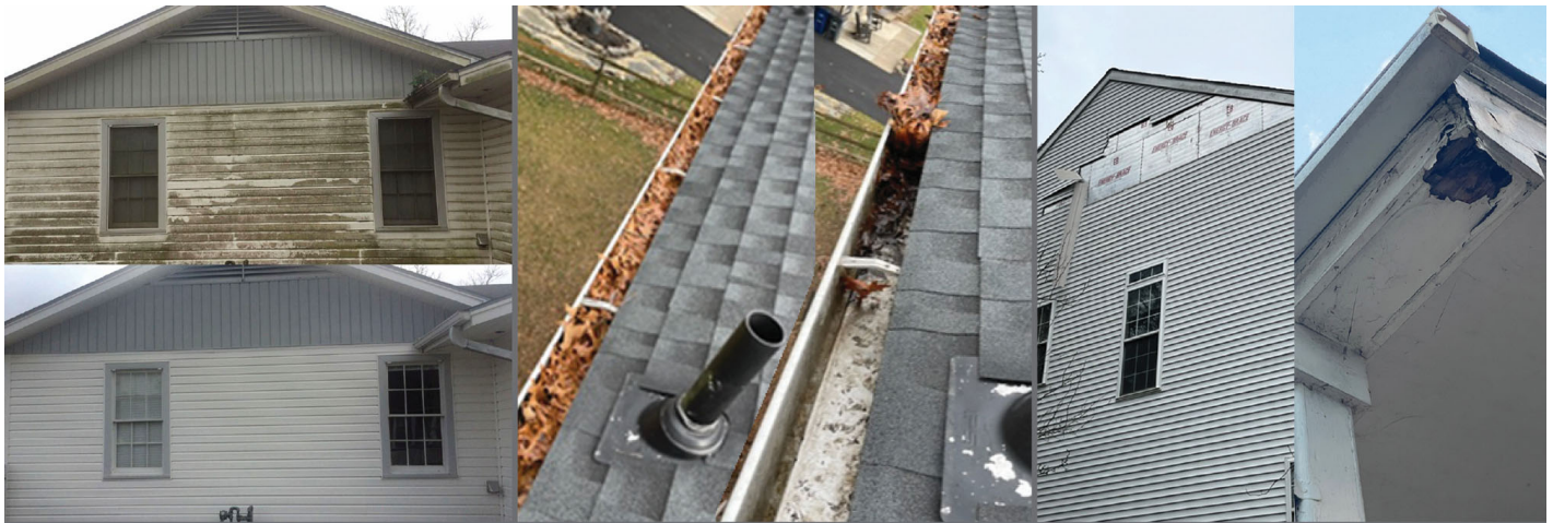
Siding & Trim Repair Rotten Wood Replacement
