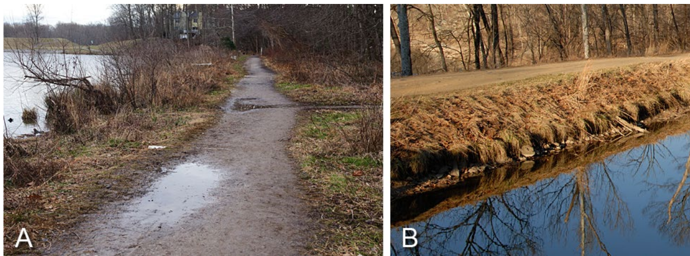
Figure 4. People love walking next to lakes and rivers. However, trails adjacent to waterways with elevations close to the normal water level end up muddy (A). The water table under the path is close to the surface. Any precipitation does not absorb into saturated soil and is unable to readily drain off the flat terrain. Four-inch PVC tubes meant to facilitate drainage are inadequate and wind up clogged. When winter arrives and the water freezes, ice expands and heaves the trail. This western section of Royal Lake's loop receives some of the most complaints about mud because it is placed in an inappropriate area, requires much upkeep, and is an unsustainable trail section. Putting the trail along the nearby slope would be a better location. Examples of sustainable, natural-surface trails next to water include the C&O Canal towpath at Great Falls National Park (B) and paths along bedrock, such as Great Falls' Billy Goat Trail (not shown).
