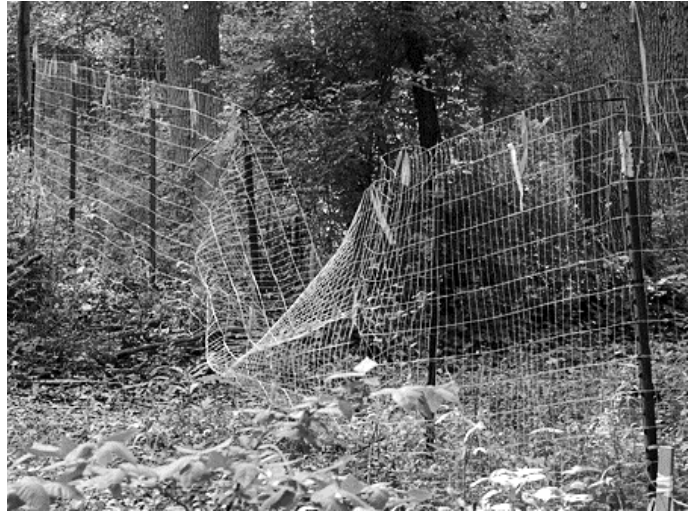
Welded wire fences encircling the LOD are to protect folks from construction activities. This example of vandalism is doubly selfish because it occurred on an unauthorized path away from the main trail.
