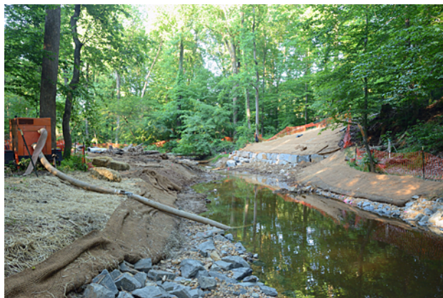
Figure 6. To temporarily reduce the creek’s water level for work on that stretch, a pump (left) bypassed water to a down-stream location. Daces and other minnows soon returned.
