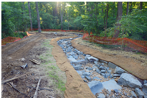
Figure 5. Near the outfall, the waterway is finished. Boulders and a curved course reduce the rushing storm water’s energy. The interim roadway (left) remained in use until completion of all major earthmoving activities.
