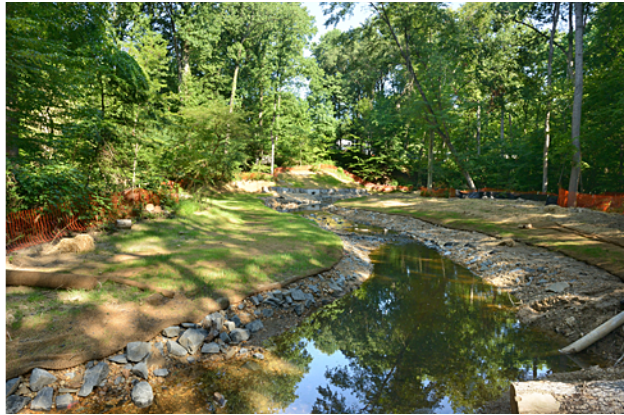
Figure 9. The preliminary work for this stream restoration is done. A shallow streambed allows water to dissipate energy across a wide surface. Grass is already sprouting along the banks. The orange work zone fence will soon come down. After adding native plants in the cool-season months, the reforestation begins—a process that continues for many decades.
