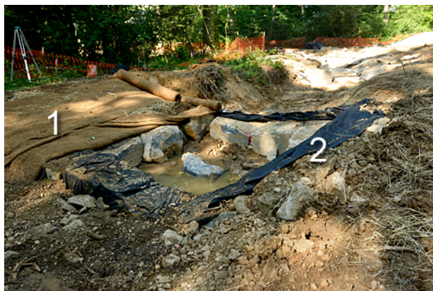
Figure 4. Restoration typically goes in a downstream direction. This incomplete section shows the coir nets (1) unrolled to retain soil. Whereas the county is moving away from plastic materials in restoration projects, synthetic geofabric (2) lines the waterway bottom with boulders and pebbles on top.
