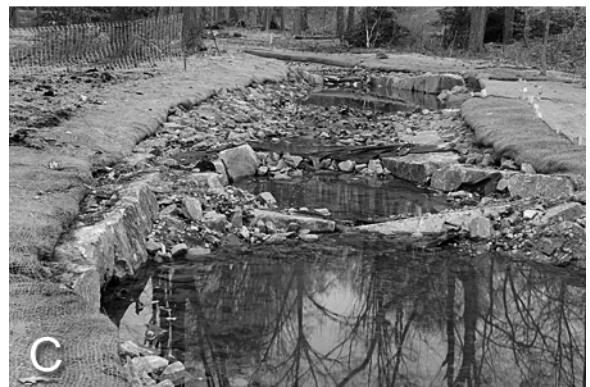
Figure 1. Indications of the surveys include (A) ribbons lining a ditch and (B) a tree tag. Stream restoration sites will look much like sections of Crooked Creek Park (C). This image of the final stages, with cooling pools and water-oxygenating cascades, shows the foundation before adding native woody plants and partial concealment by foliage.
